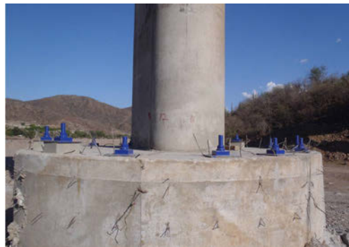
Self-drilling anchors, Batopilas Bridge - Mexico
