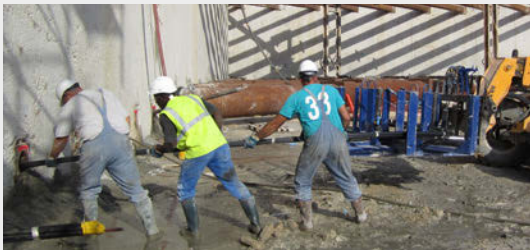
Strand anchor uncoiler
