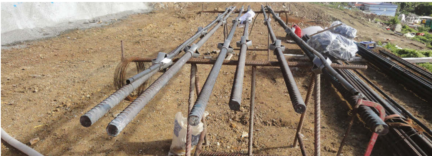
Preparation of Freyssi500 soil nails - Martinique, France
