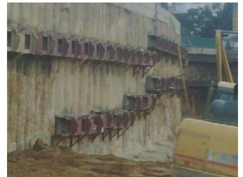
Temporary strand anchors - Bangalore Metro - India
