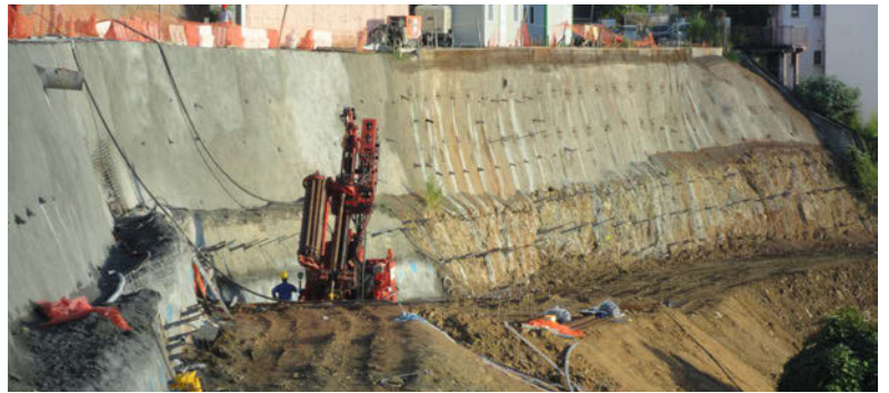
Freyssi500 soil nails - Morne Calebasse - France
