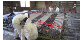
Production of permanent Freyssibar anchors
