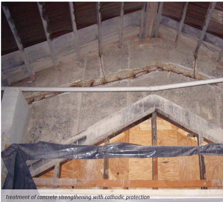
Strengthening with TFC
