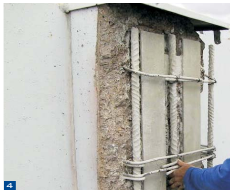
1 / Facade repair 2 / Resealing joints 3 / Facade repair access system 4 / Forming concrete repair 5 / External post-tensioning
