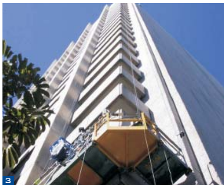
1 / Facade repair 2 / Resealing joints 3 / Facade repair access system 4 / Forming concrete repair 5 / External post-tensioning
