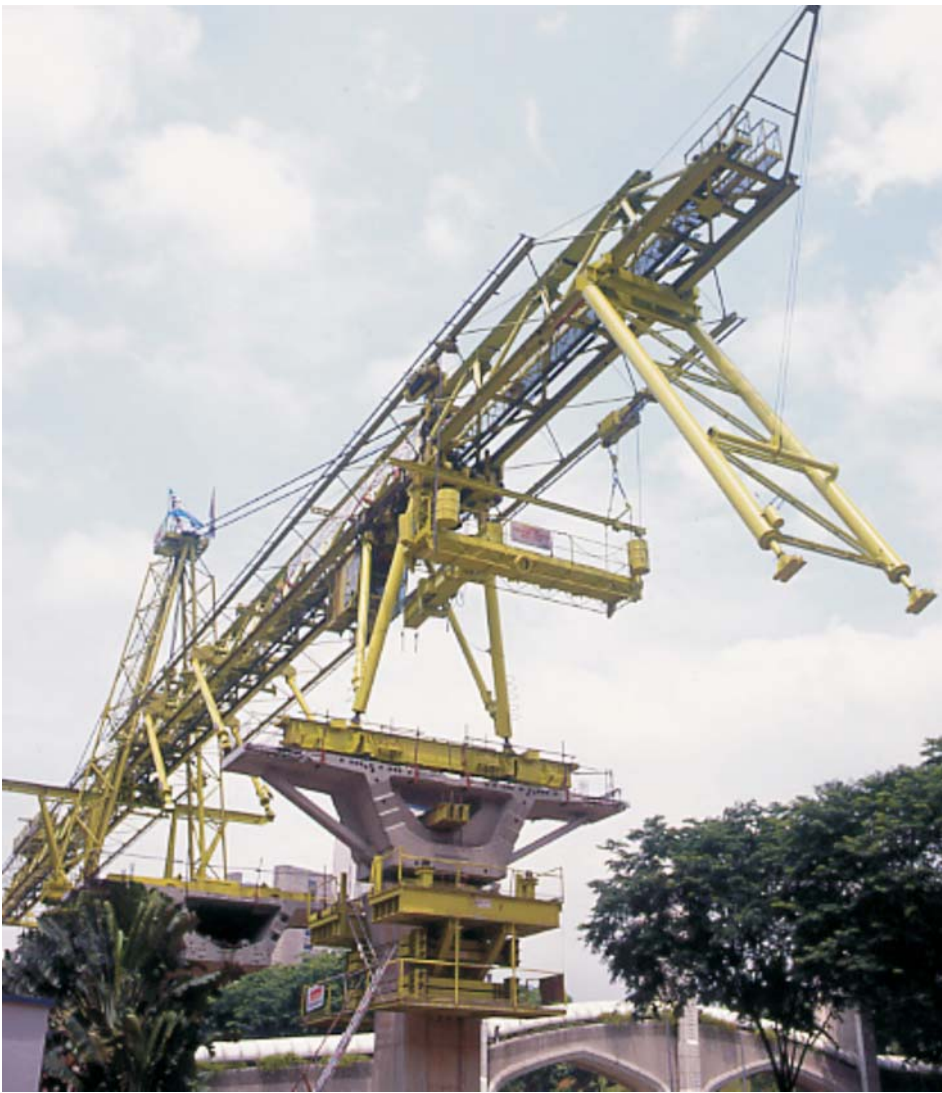
Kuala Lumpur LRT: launching over pre-installed pier segment
