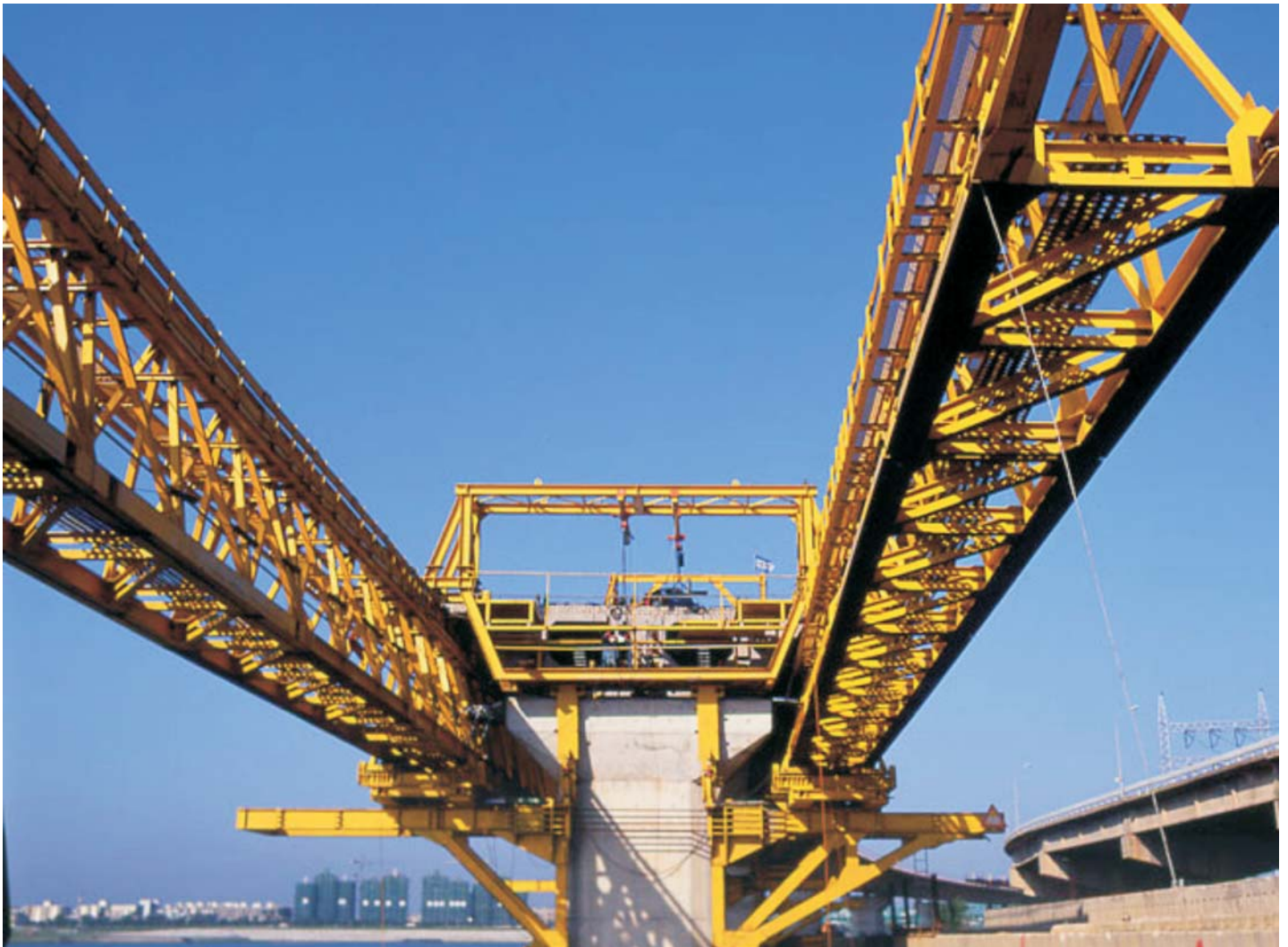
Riverside IV, Korea: assembly truss and pier bracket
