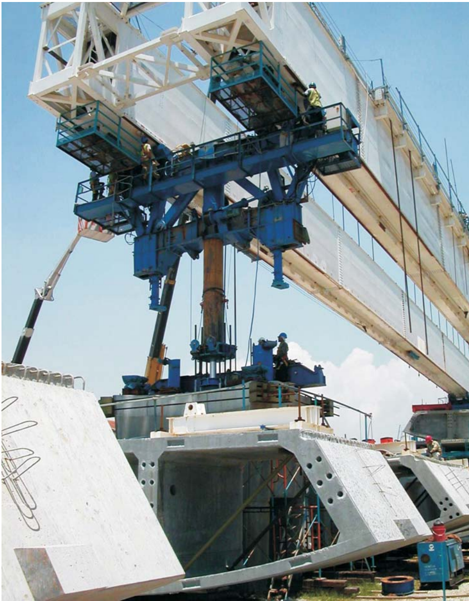
Sungai Prai: launching gantry auxiliary front support, segments waiting for lifting
