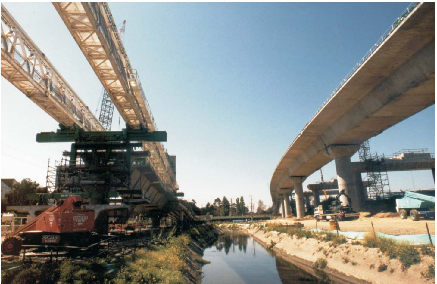
Western Link: Left, ramps erected with overhead gantry. To the right, main line half erected
