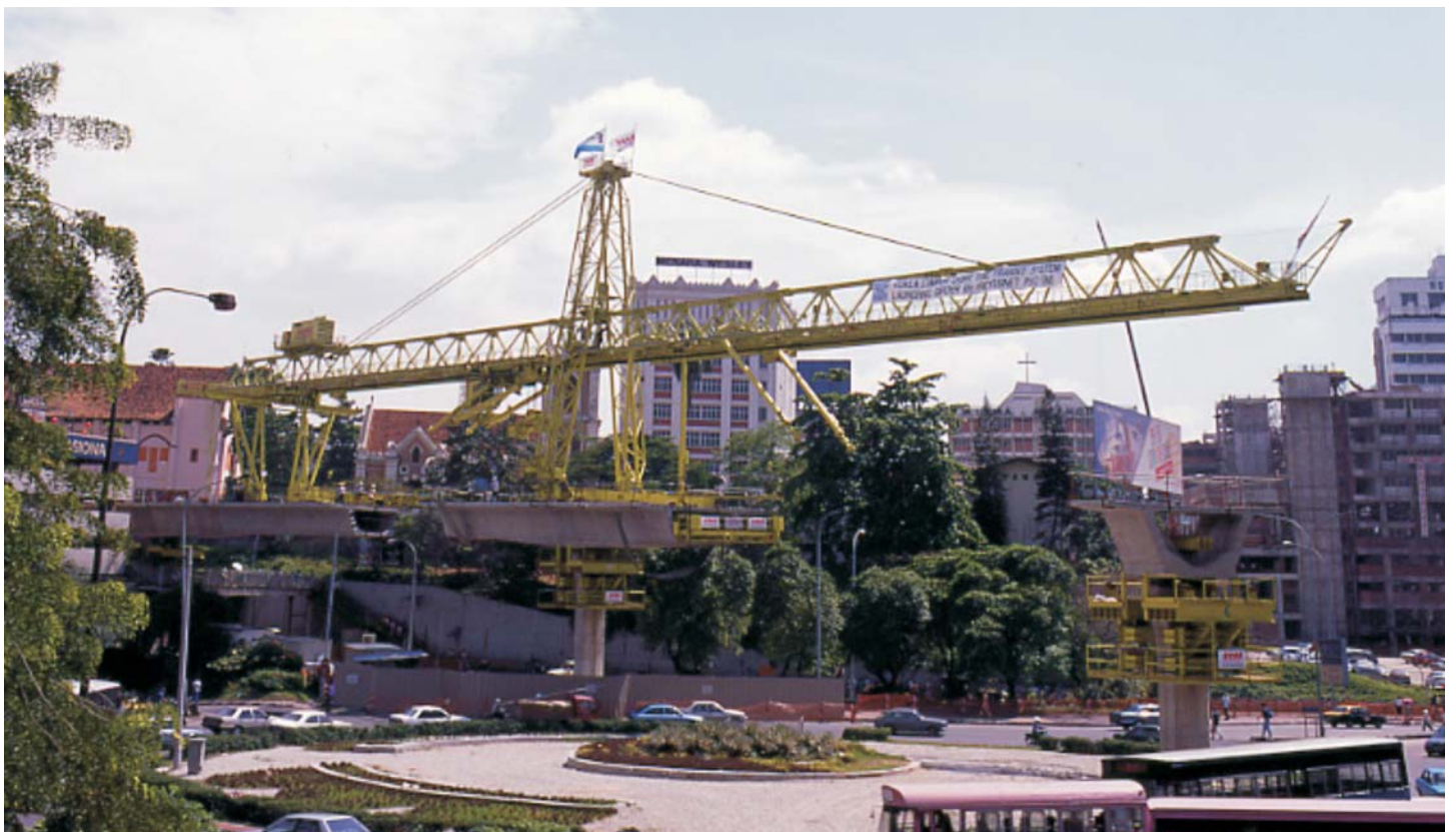
Kuala Lumpur LRT: cantilever erection in progress
