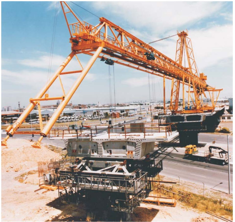
Westgate Freeway: pier segment placing
