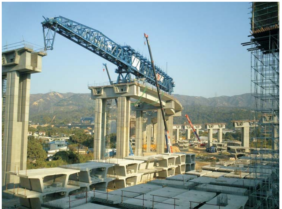
Deep Bay Link: launching of truss
