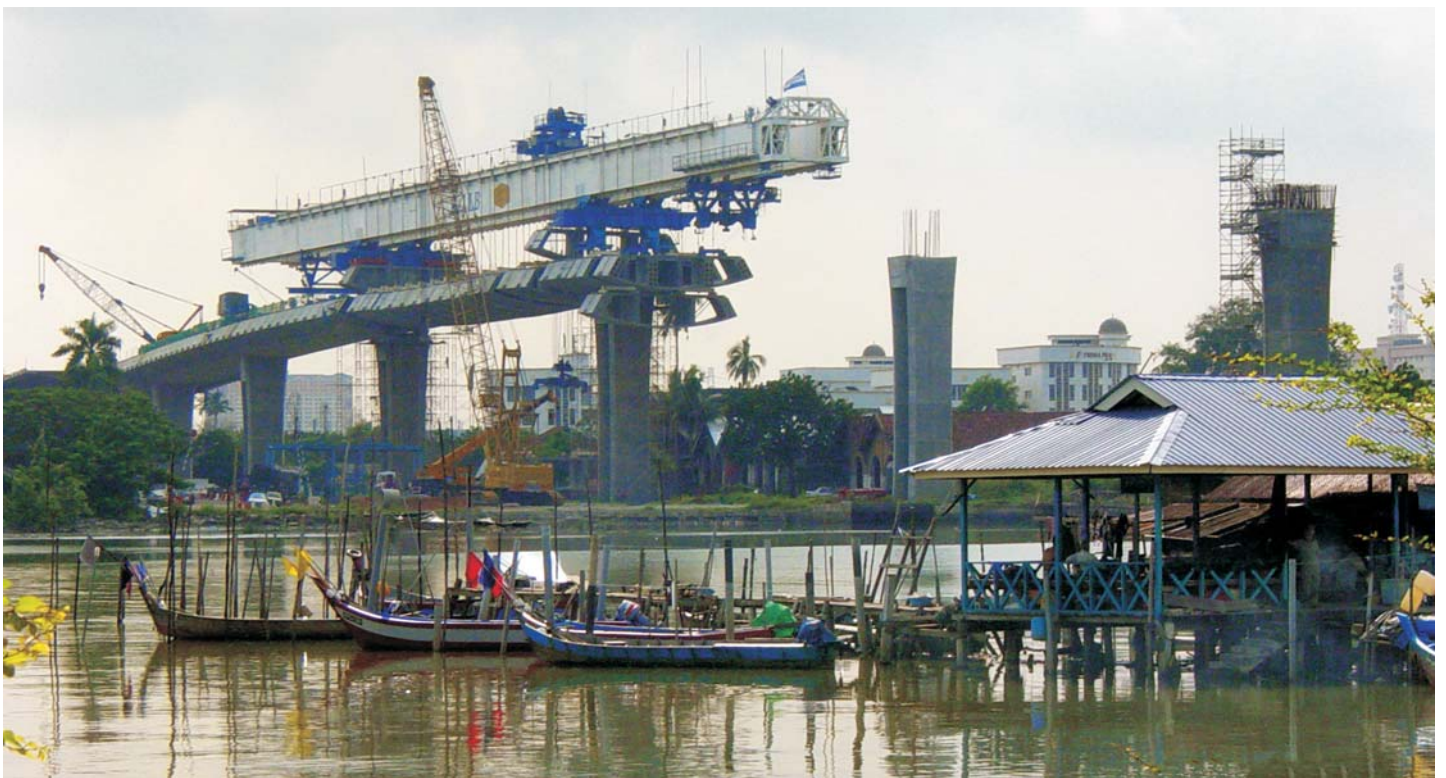
Sungai Prai: full span supported by the gantry
