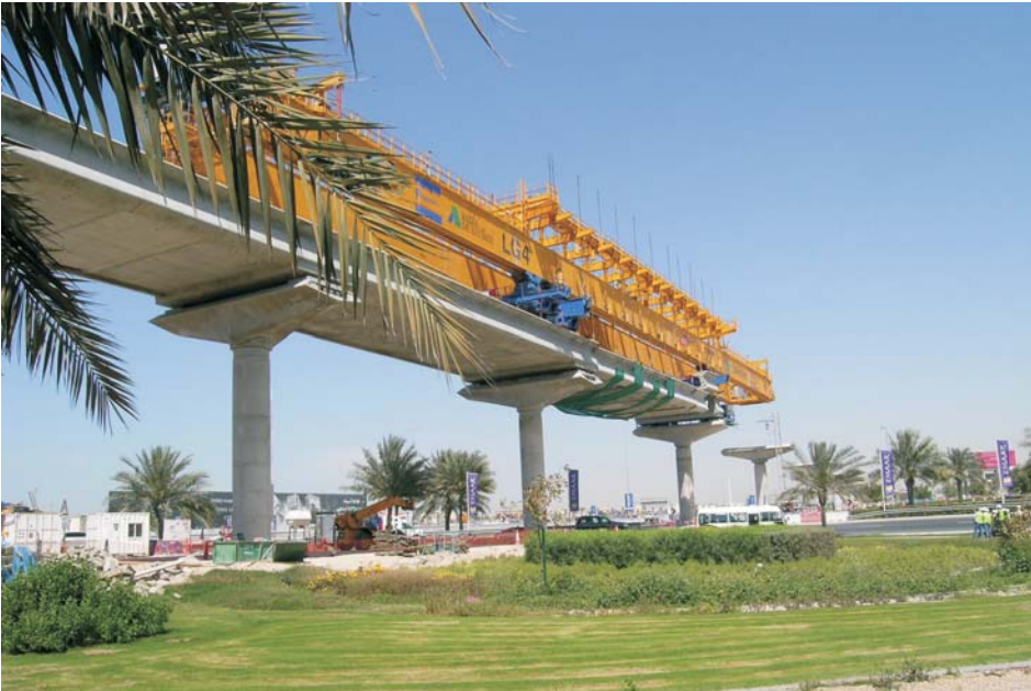
Dubai LRT: span finishes prior to launching
