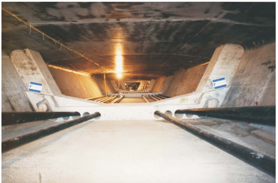
Western Link external post-tensioning
