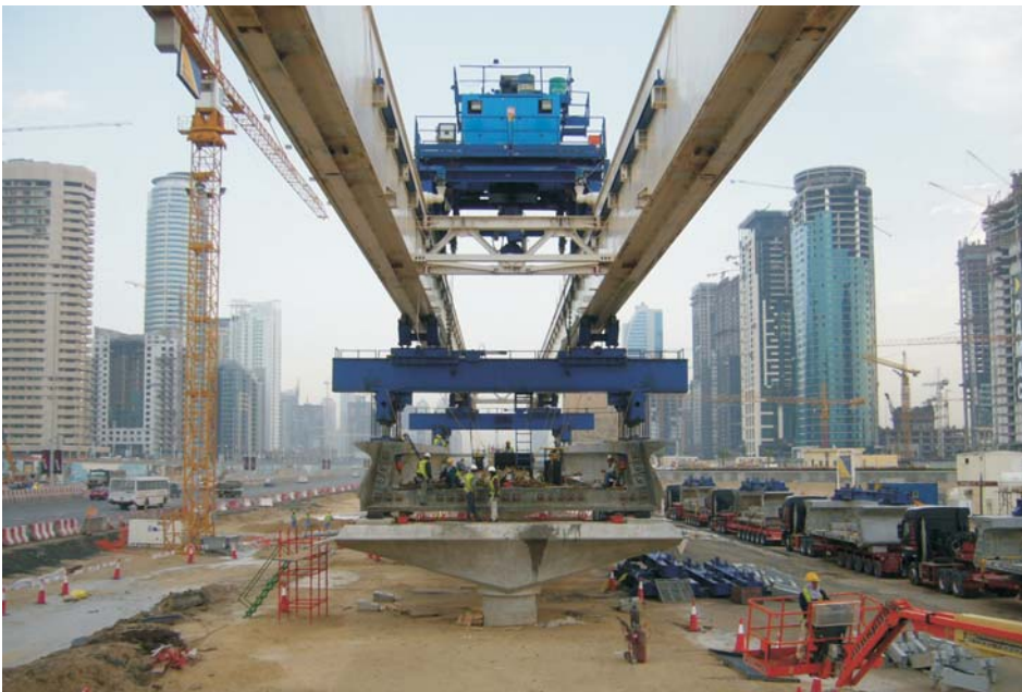
Dubai LRT: connection of segments to the launching gantry
