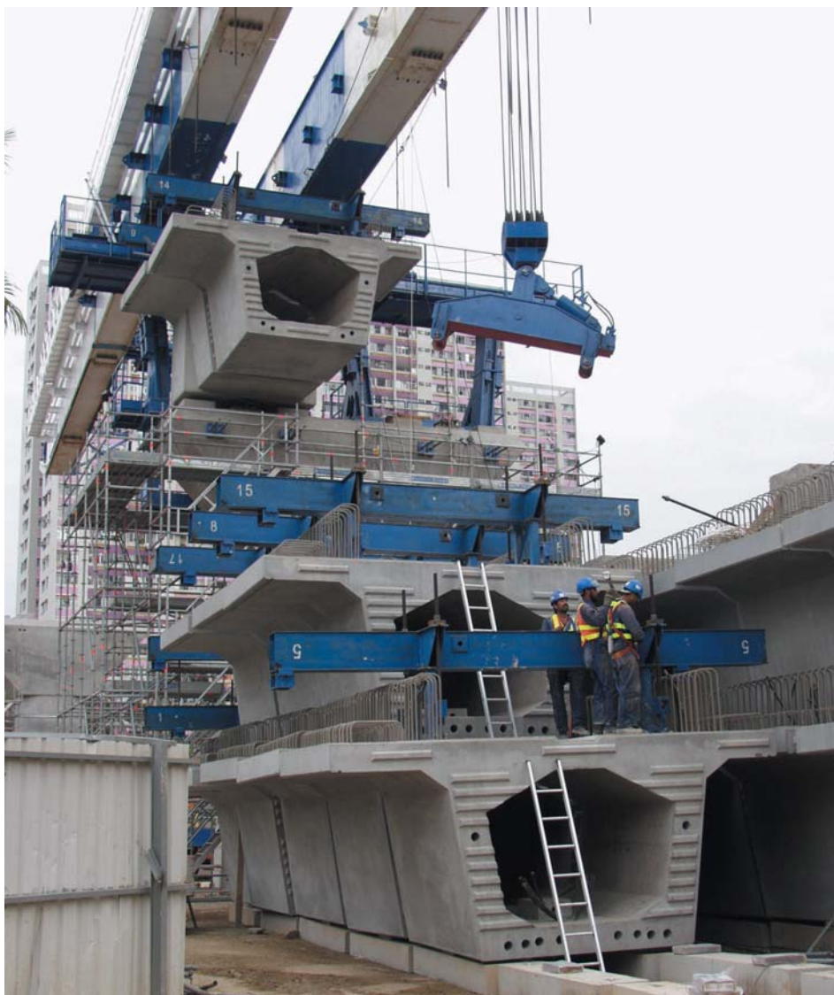
East Rail: lifting of segments
