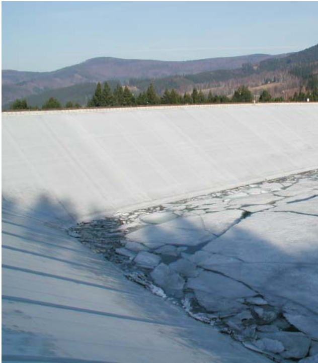
▲ Moravka Dam, Czech Republic: Exposed PVC geomembrane to rehabilitate an embankment dam with bituminous concrete facing
