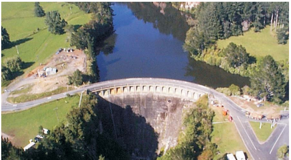
► Arapuni Dam, New Zealand: Fissure grouting and jet grouting
