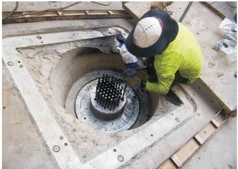
▼ Wivenhoe Dam, Australia: 61 strand anchor head
