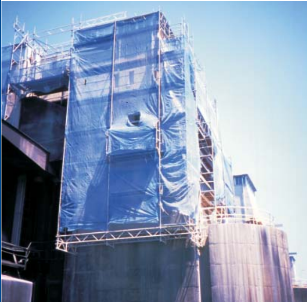
▲ Pouzin Dam, France: Treatment of the corroded reinforcement steel
