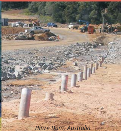
Hinze Dam, Australia
