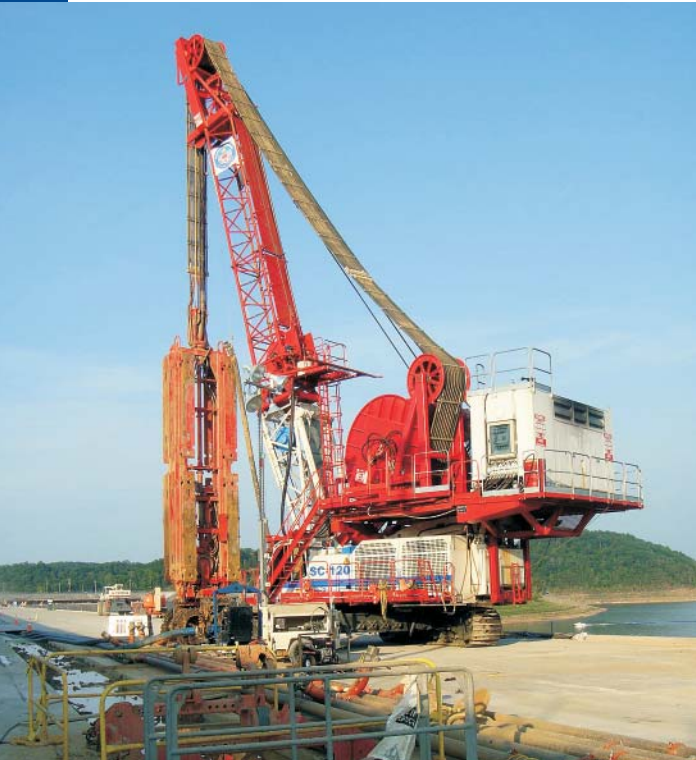
▲ Wolf Creek, Kentucky USA: Hydroraise ready to start cut-off wall excavation
