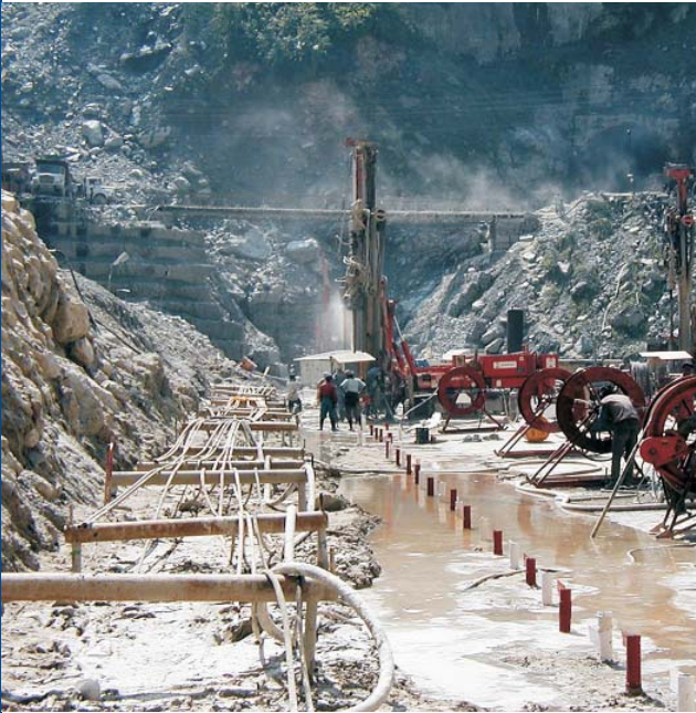
▲ Teesta Dam, India: Jet grouting and grout injection
