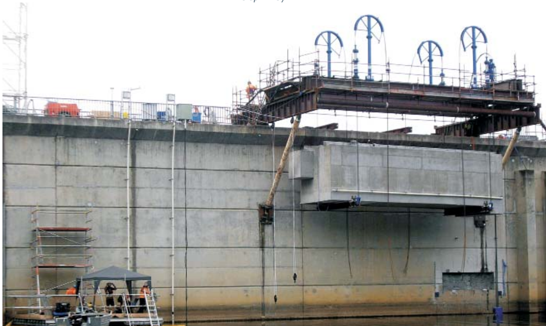
▼ ▲ Tallowa Dam, Australia: Installation of a fish lift with strand lifting jacks
