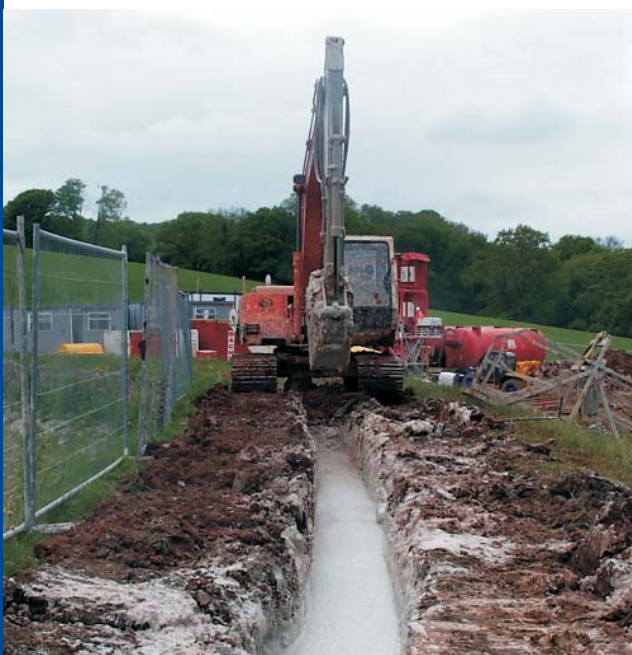
▲ Leigh Reservoir, United Kingdom: Cement bentonite cut off barrier installed from the dam crest
