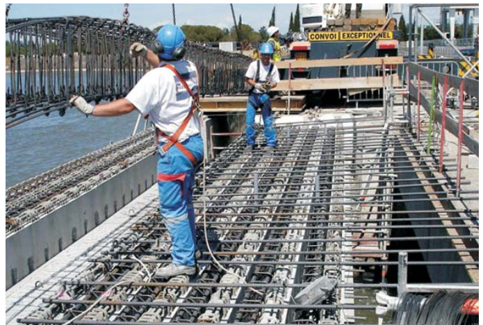
▲ Vallabregues Dam, France: Removal and replacement of a bridge over a spillway
