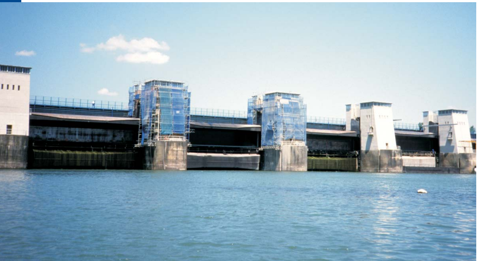
▼ Pouzin Dam, France: Repair of the concrete with anti carbonation coating
