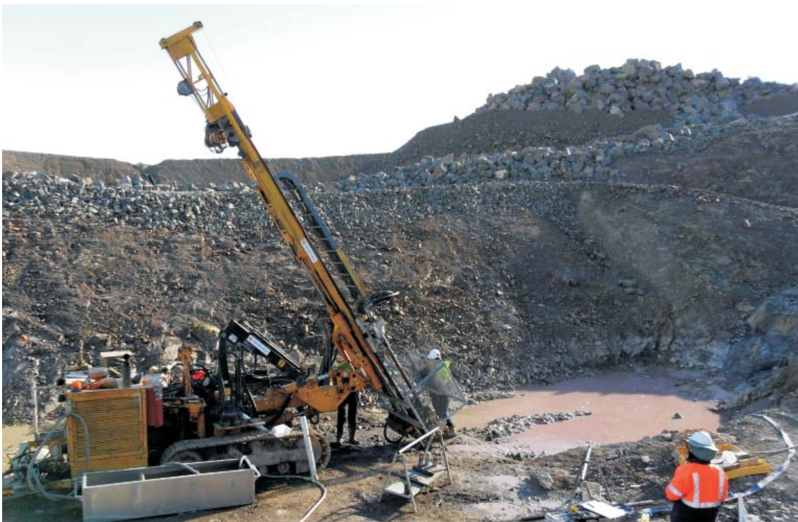
◀ Cotter Dam, Australia: GIN grouting
