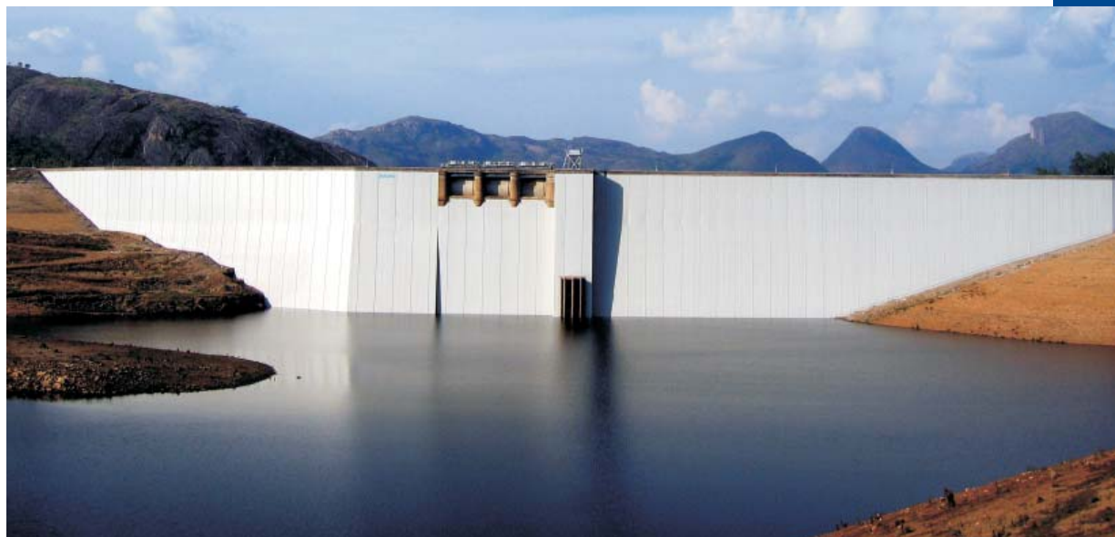
▶ Kadamparai Dam, India: Exposed PVC geomembrane to rehabilitate a 67m high masonry dam
