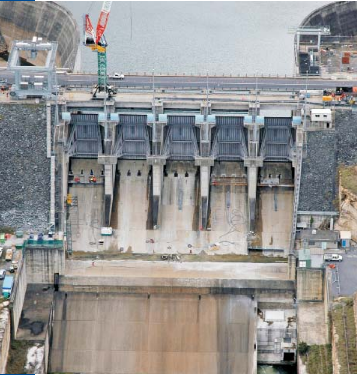
▲ Wivenhoe Dam, Australia: Spillway stabilisation with large capacity rock anchors
