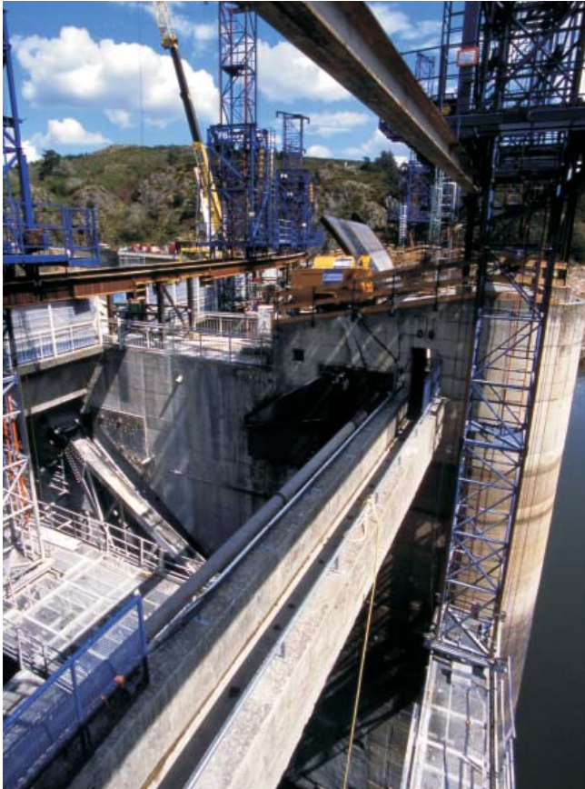
▼ ▲ Grangent Dam, France: Dewatering and repair of radial gate lower anchors with new tie rods, including provision of mast climber access
