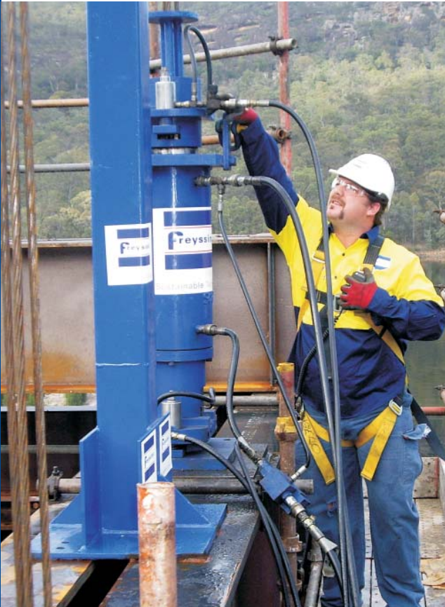
▼ ▲ Tallowa Dam, Australia: Installation of a fish lift with strand lifting jacks
