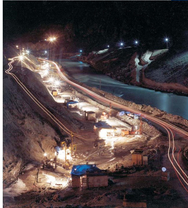
▲ Clyde Dam, New Zealand: Stabilisation of a rock slope by grouting on left bank of dam using permeation grouting.
