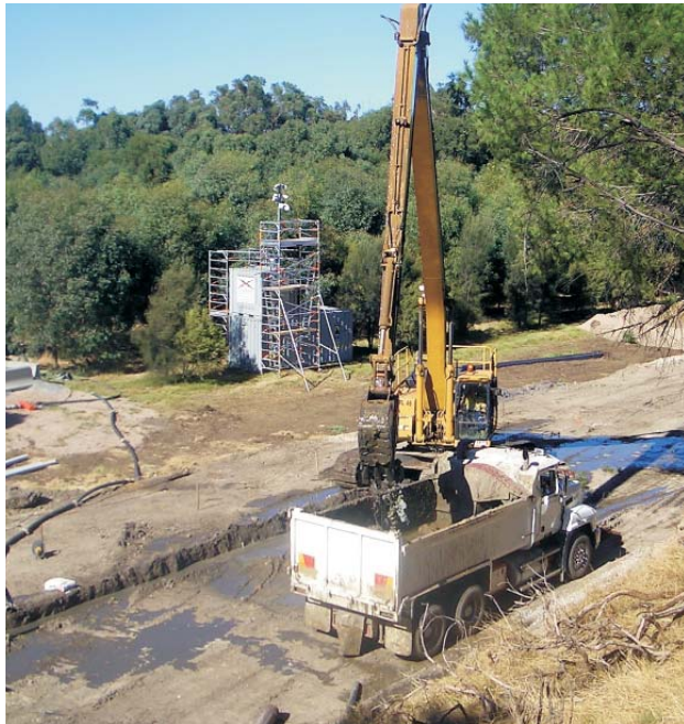
Permeable barrier collector drain excavated under biopolymer. First used in Australasia at Hays Creek Dam in New Zealand
