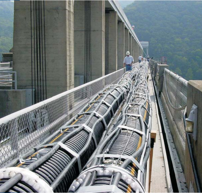
▲ Bluestone Dam, USA: Large capacity prefabricated 61 strand anchors
