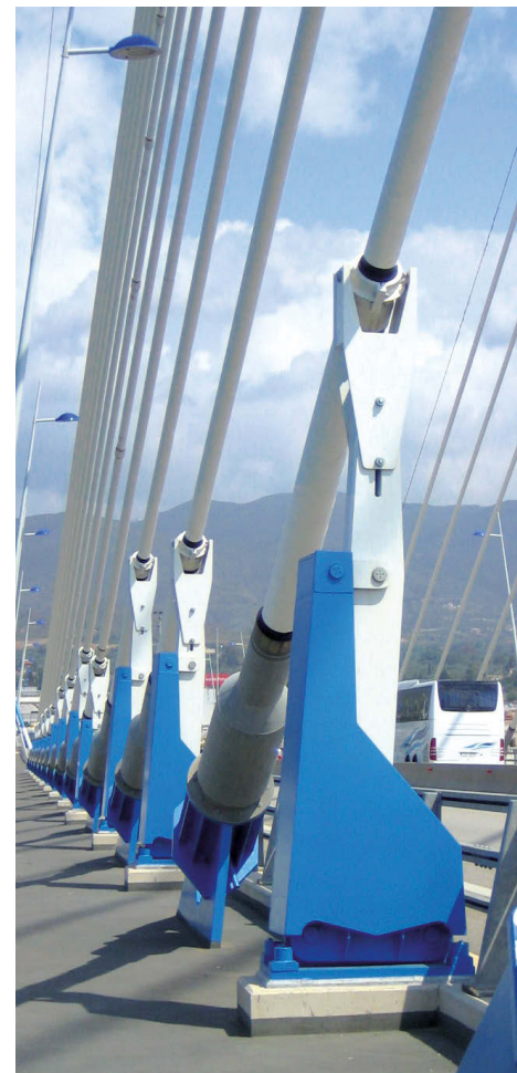
PED damper Charilaos Trikoupis bridge / Greece
