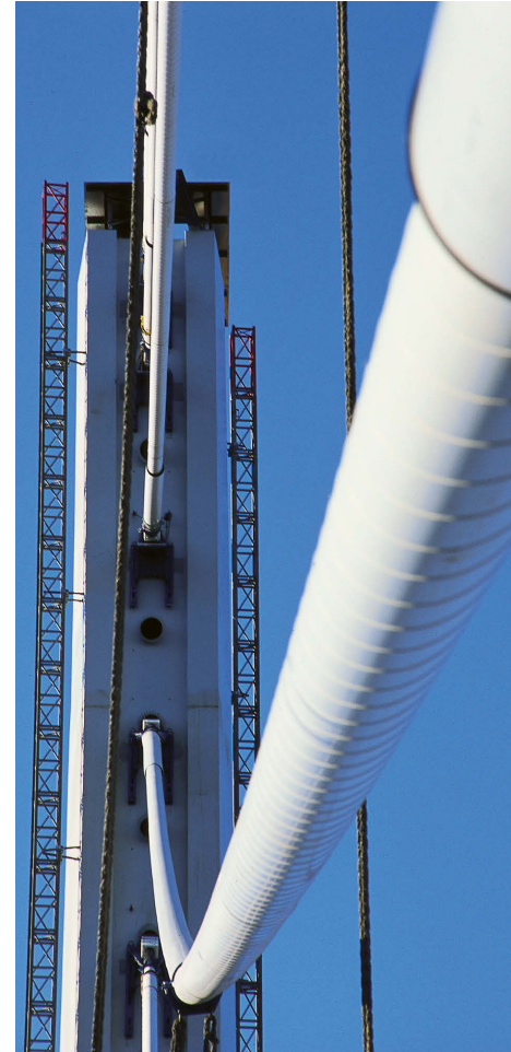
Helical fillet Millau bridge / France
