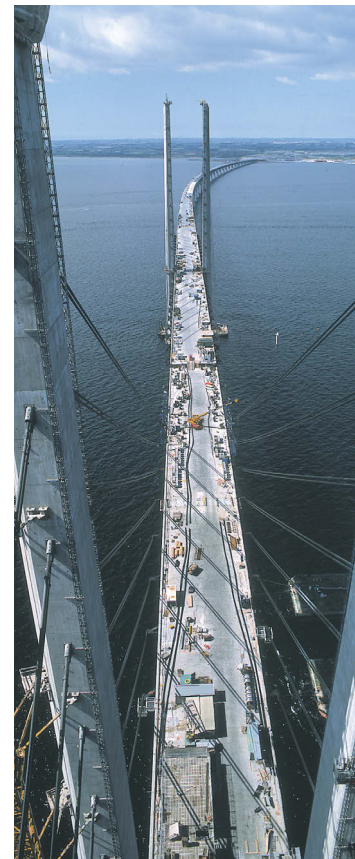
Øresund bridge Denmark-Sweden
