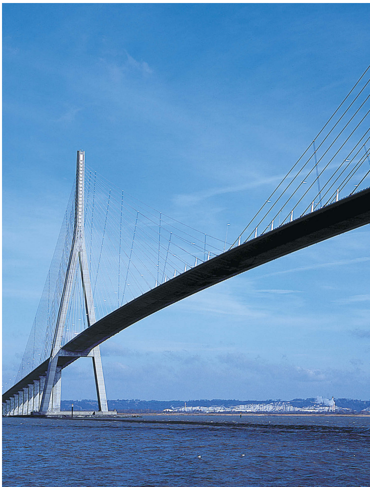
Normandie bridge cross tie / France
