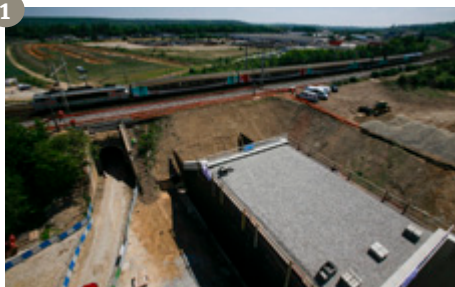
1 - Prefabricating the structure next to the track and positioning the driving nose
