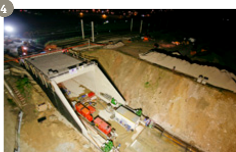
4 - Final sliding and backfilling
