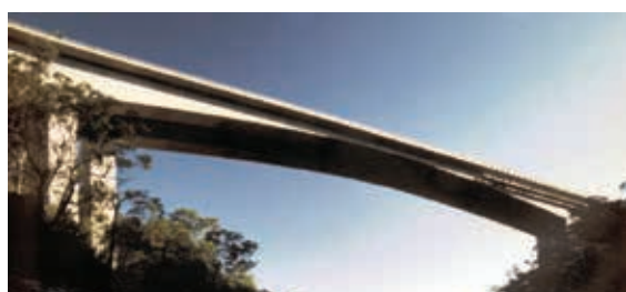
External post-tensioning with greased and sheathed strands, Pheasants Nest Bridge, Australia
