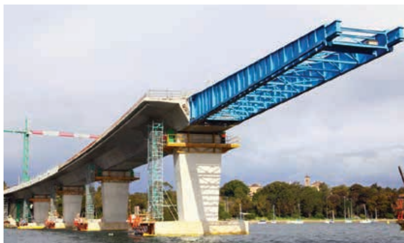
Iron Cove Bridge, Sydney, Australia
