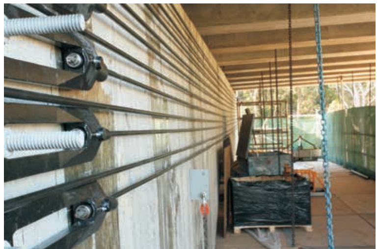
Pier headstock strengthening, M2 Upgrade, Sydney, Australia
