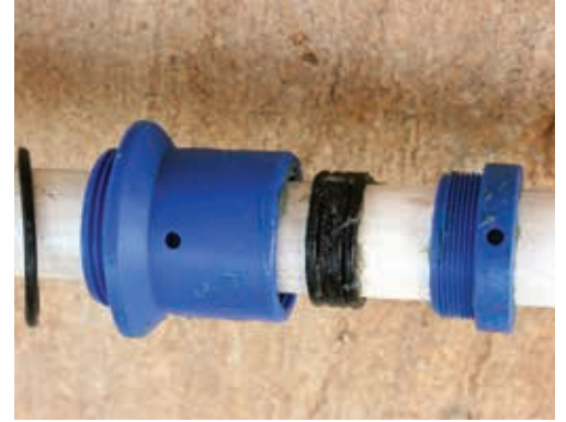
Plastic fittings to seal the outer HDPE duct
