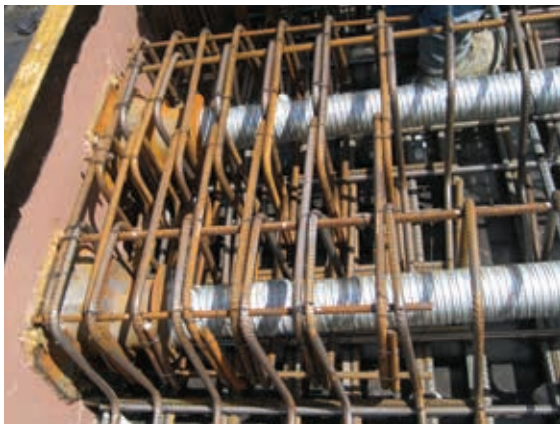
Example of anti-burst reinforcement
