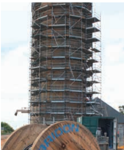
Underbool Grain Silos strengthening, Australia
