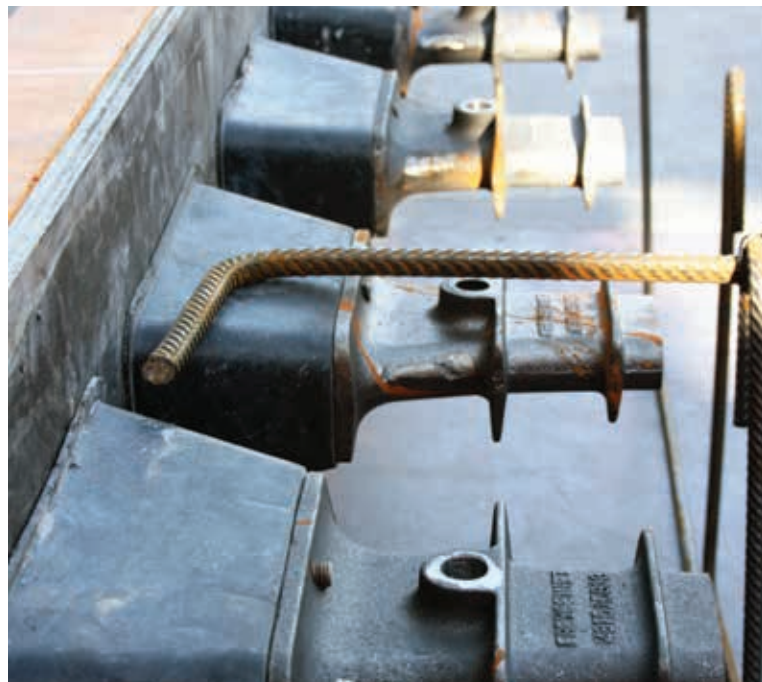
S Range anchorages prior to placing concrete
