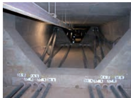
HDPE ducts for external prestressing
