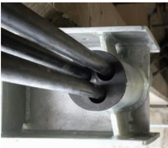
Multitube deviation saddle
