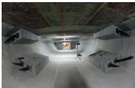
Internal bonded prestressing, blisters for tendon lapping
