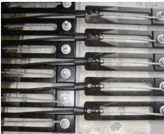
Live ends before stressing
