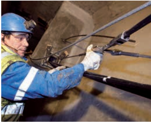
Greased and sheathed strands being winched through
