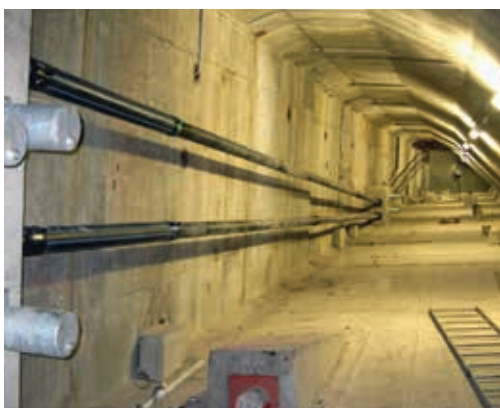
External prestressing, West Gate Bridge, Melbourne, Australia
