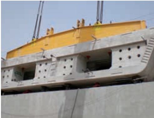
Lifting : prestressed connection between a segment and a beam.
