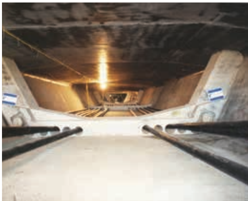
External prestressing, Western Link, Melbourne, Australia
