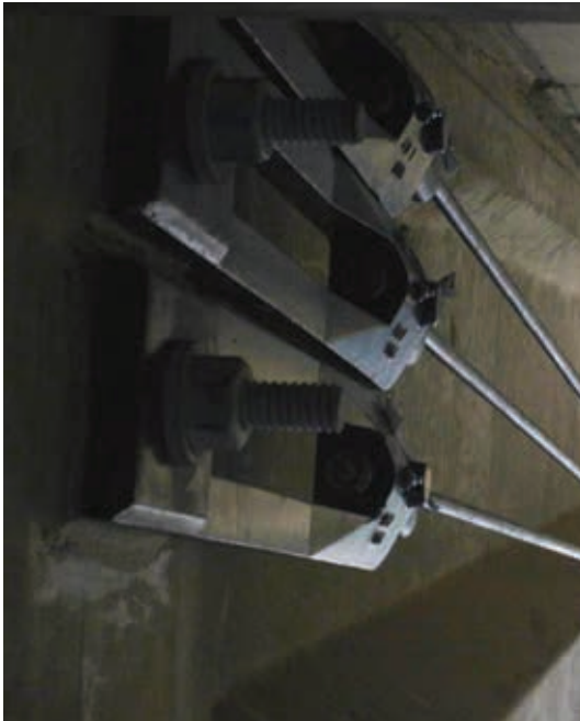
1R15 anchorages stressed
