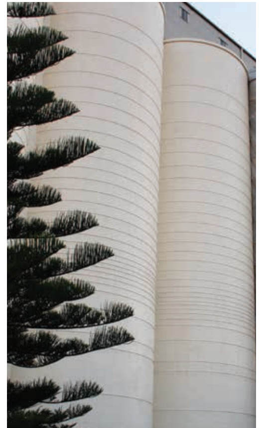
Geraldton Grain Silos, Australia
