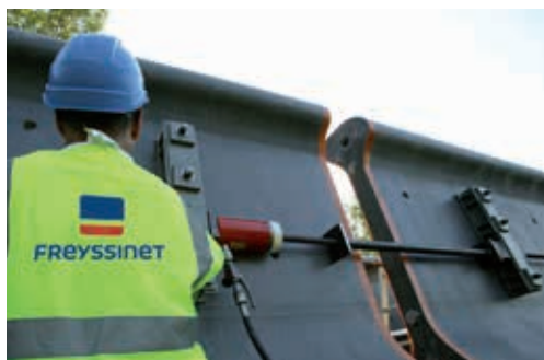
Precast segments assembly
