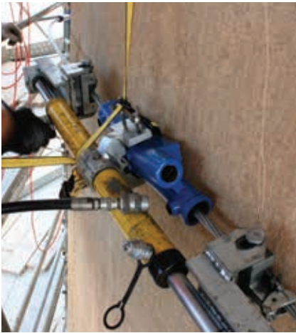
1x15 Anchorage, Underbool Grain Silos, Australia
