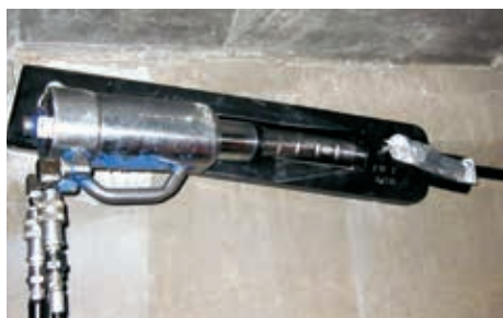
Stressing of the 1R15 anchorage with curved nose and monostrand jack
