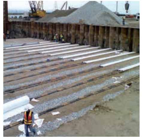
Permanent ties for quay walls
