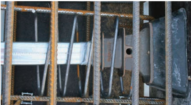
S Range anchorages anti-burst reinforcement
