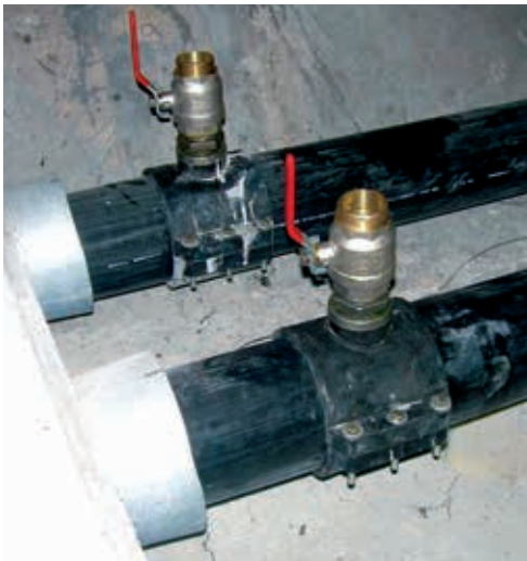
Injection inlets on HDPE pipes
