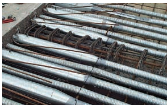
Coupler cover installed
