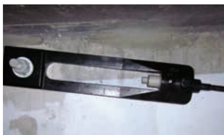
1R15 anchorage in final configuration
