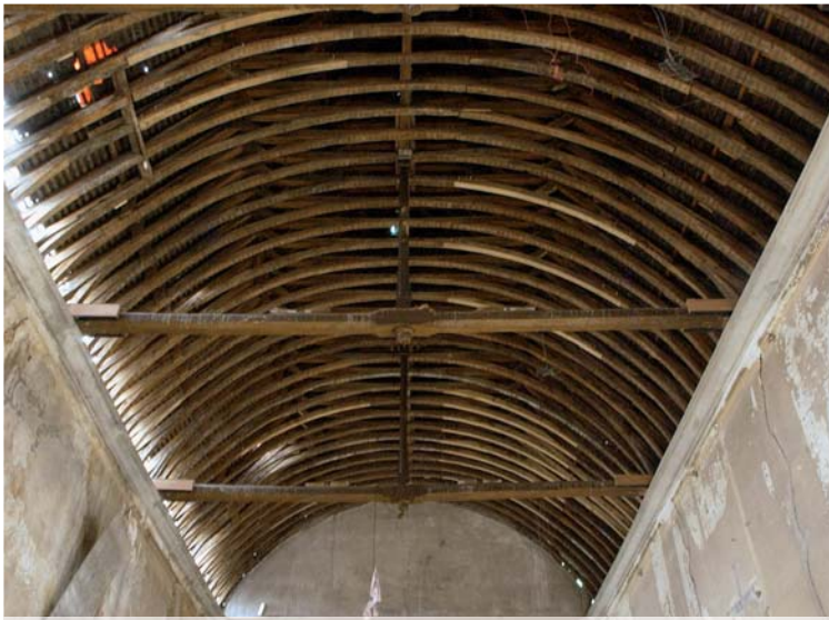
Repair of curved vaulted timber frame tie beams
