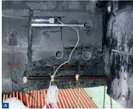
1 /Impressed Current Cathodic Protection on steel wharf structure 2/Concrete repair 3/Carbon fibre installation 4/Impressed Current Cathodic Protection installation 5/Strengthening of a silo
