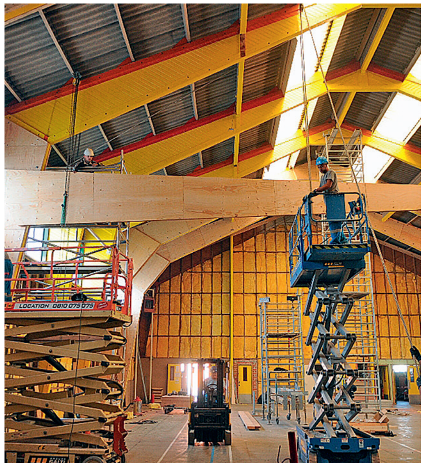
Timber frame splinting
