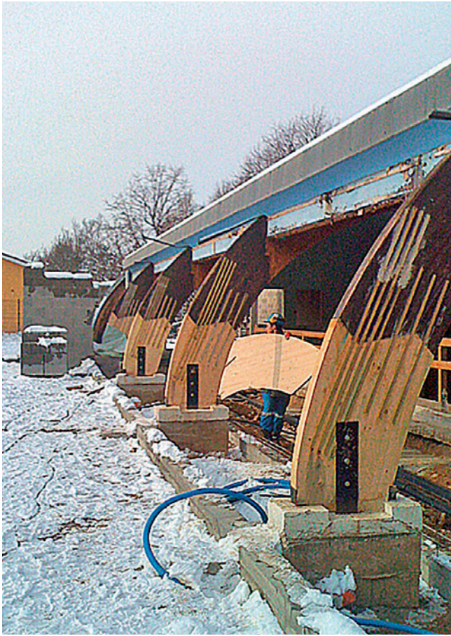
Installing new timber using scarf joints
