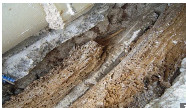
1 - Beam broken due to mechanical failure
