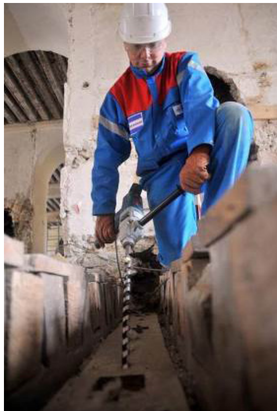
Reinforcing a beam by adding a resin concrete reinforcement Drilling recesses for the tie rods
