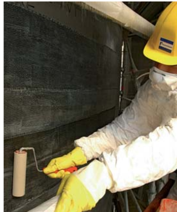
Strengthening metal tank for earthquakes with Foreva® TFC
