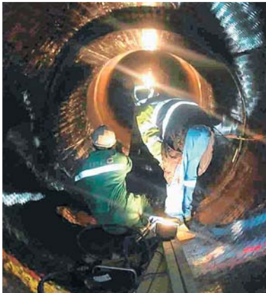
Repair of walk through drinking water pipe with HDPE liner
