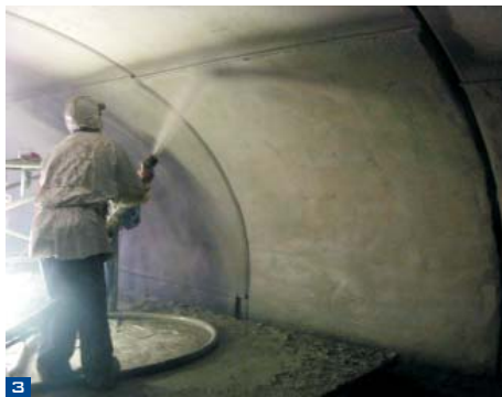
1/Earthquake strengthening of reservoir 2/Earthquake strengthening of reservoir 3/Culvert shotcreting 4/Reservoir roof replacement 5/Sewer manhole coating
