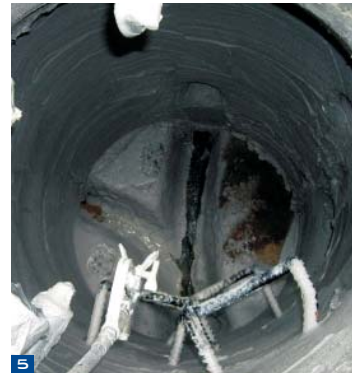
1/Earthquake strengthening of reservoir 2/Earthquake strengthening of reservoir 3/Culvert shotcreting 4/Reservoir roof replacement 5/Sewer manhole coating
