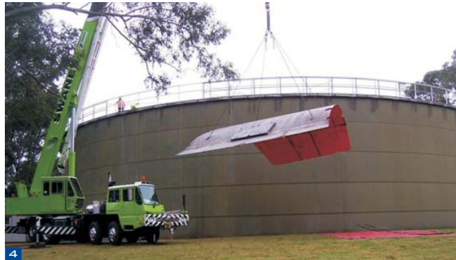
1/Earthquake strengthening of reservoir 2/Earthquake strengthening of reservoir 3/Culvert shotcreting 4/Reservoir roof replacement 5/Sewer manhole coating
