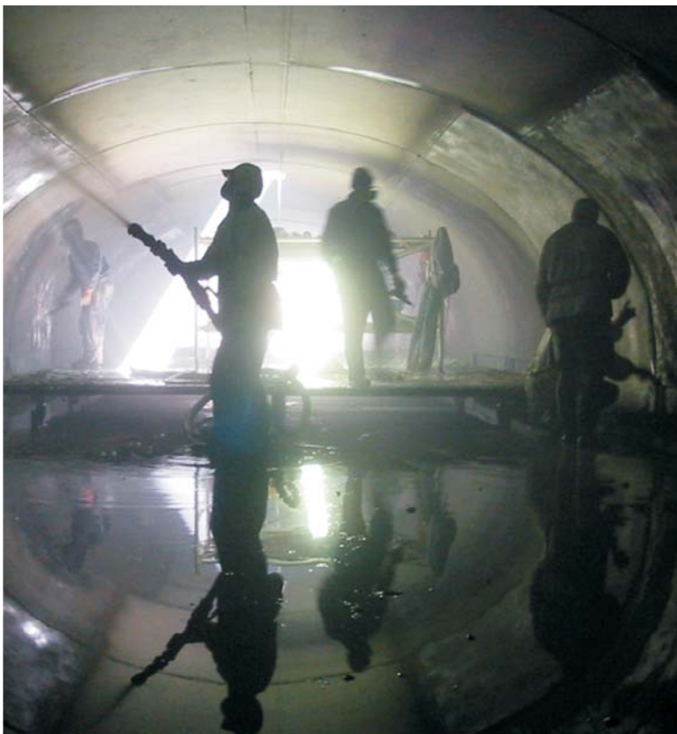
Culvert wall strengthening with shotcrete
